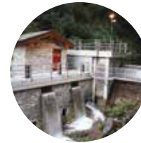
HYDRO POWER PLANTS
